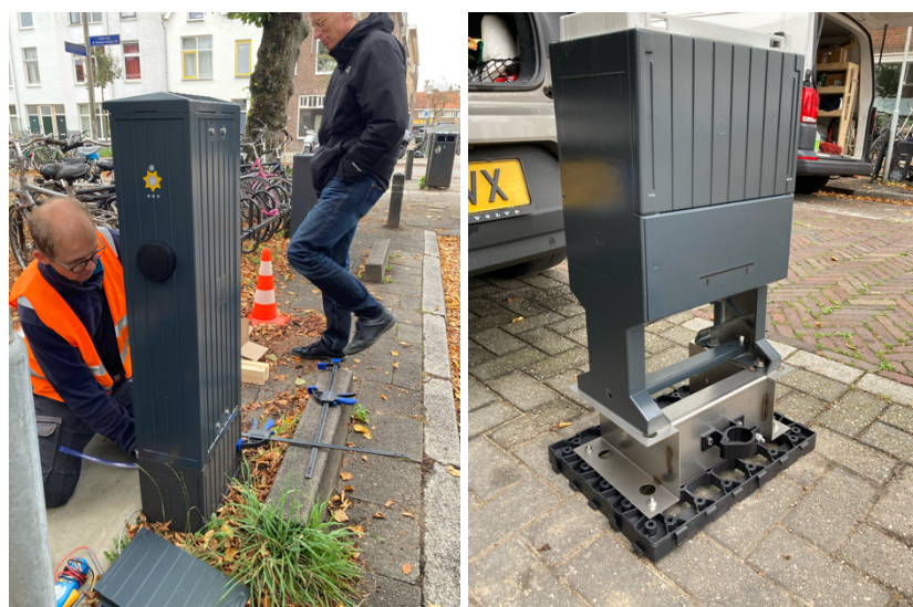
Figure 24: We Drive Solar V2G charger installation
